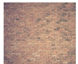
Duvari Zid Wall
